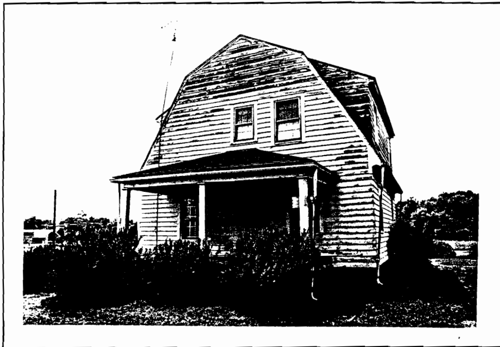
Figure 87: House at 5215 Plank Road (88-282)
