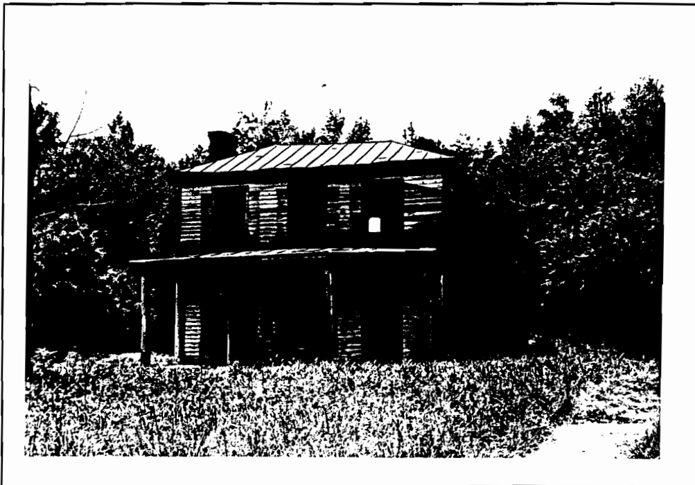
Figure 84: House on Jefferson Davis Highway (88-10)
