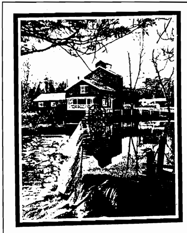
Figure 67: Historic Photograph of Stanard's Mill (88-24)
